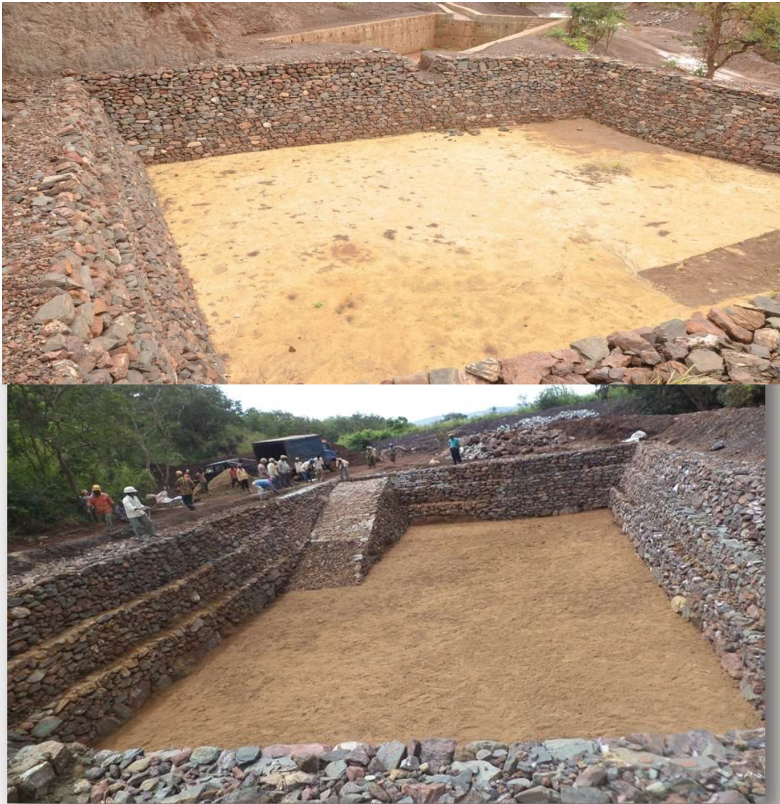
Rainwater harvesting pit at Neerlabbi pit
