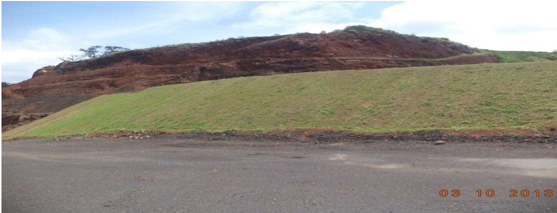
Geo-coir mats put on waste dump terrace at Dabaxikolla Pit
