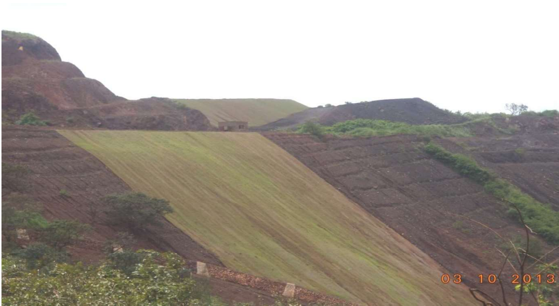
Geo-coir mats layed on dump terrace at Dabaxikolla Mine Pit
