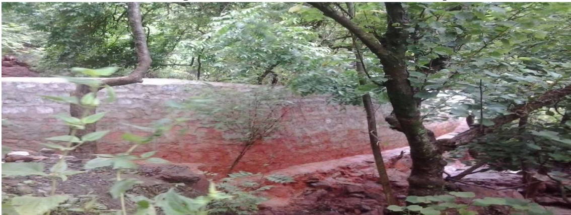
Stone masonry check dam constructed at Neerlabbi Mine Pit
