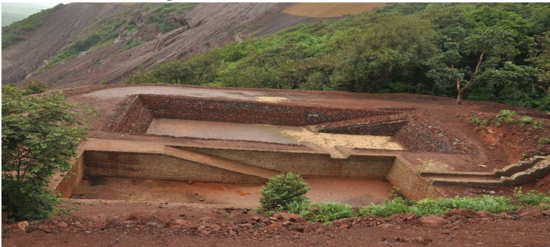
Silt Settling tank constructed in Dabaxikolla Mine pit
