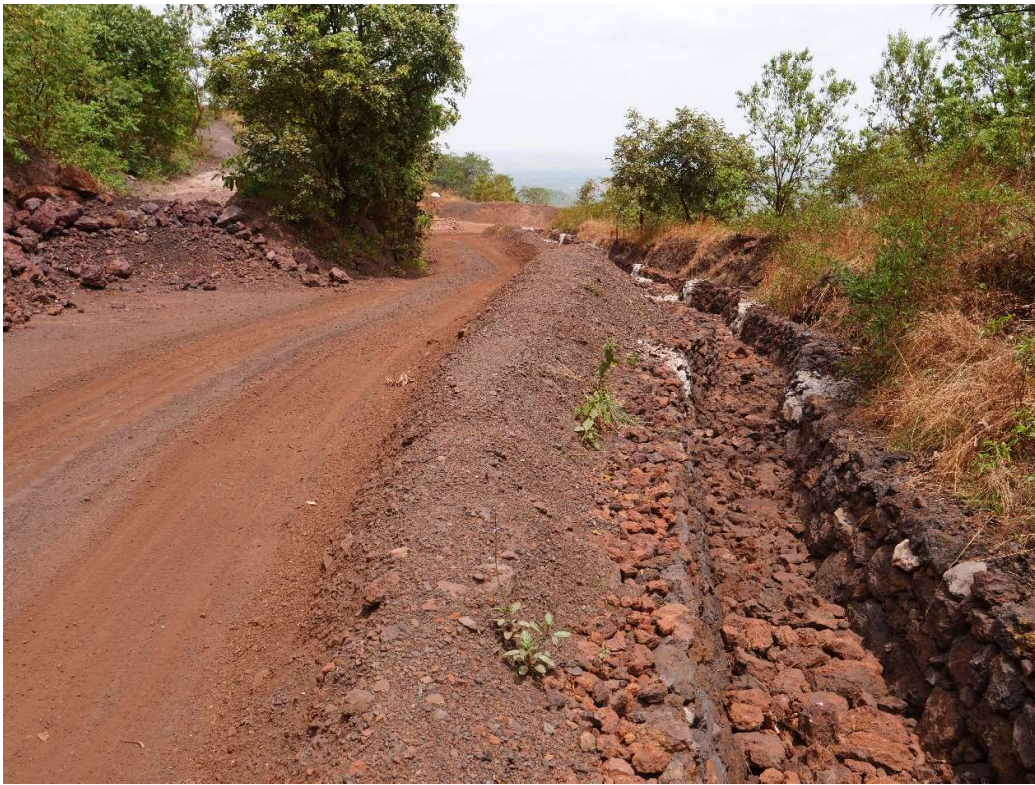
Garland Drain constructed during the Year 2022-23 measuring 50 meters
