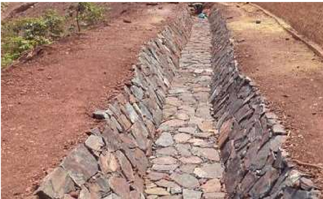
Garland Drain constructed below toe of the dump for rainfall runoff water
