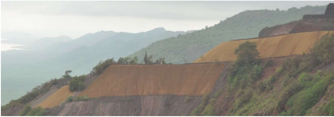
Terracing and Geo-coir mats layed on the dumps at Governor Point
