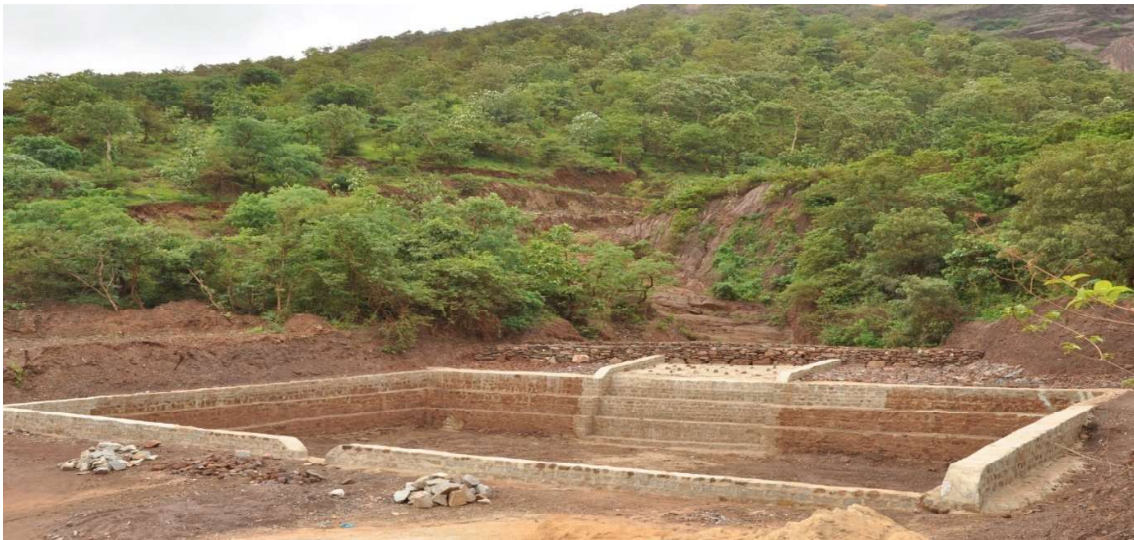
Silt Settling tank constructed outside the mine lease area
