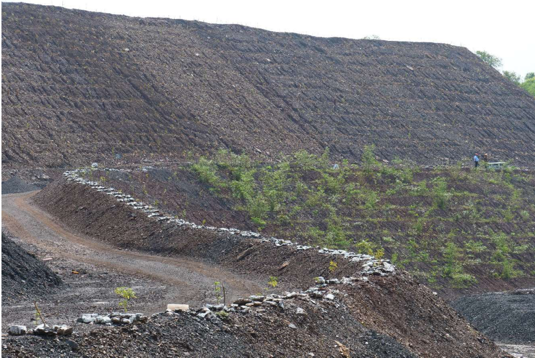
Systematically terraced dump at Dabaxikolla
