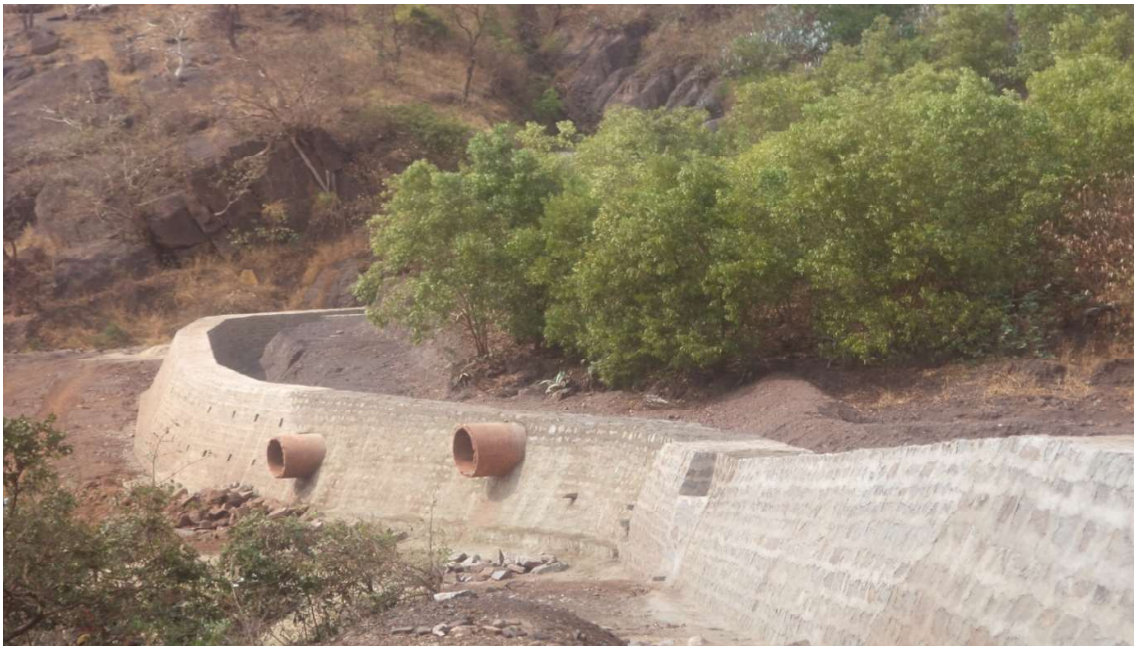
Masonry toe wall constructed at toe of waste dump with weep holes
