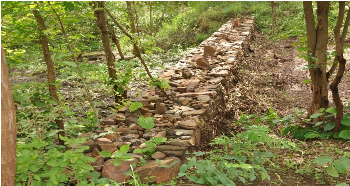
Loose boulder check dam constructed within the mine lease
