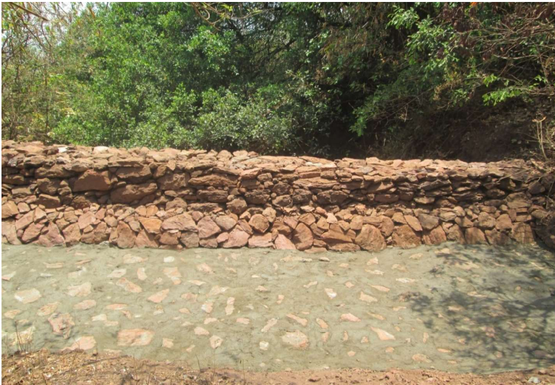
Loose boulder check dam constructed within the mine lease
