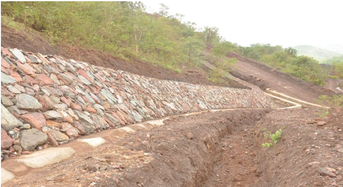
Dry Stone Retaining wall constructed for D1/13 dump at Ramghad
