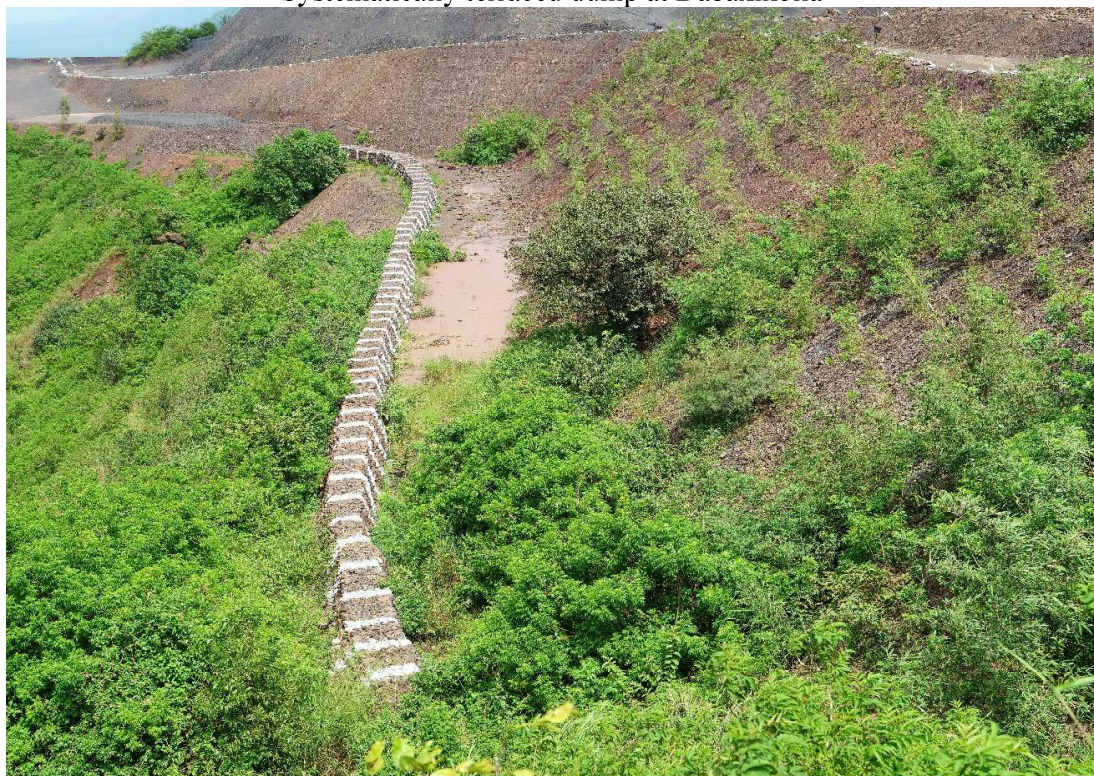
Toe Wall constructed for Surface Dumping
