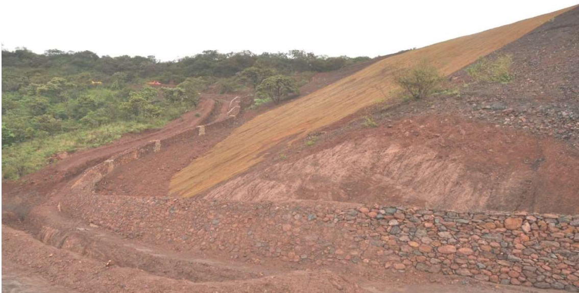
R&R Dry Stone Wall constructed below toe of waste dump in Ramghad
