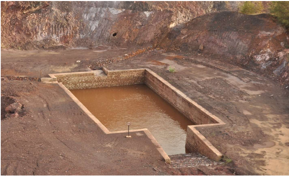
Silt Settling tank constructed at Governor Point Mine pit
