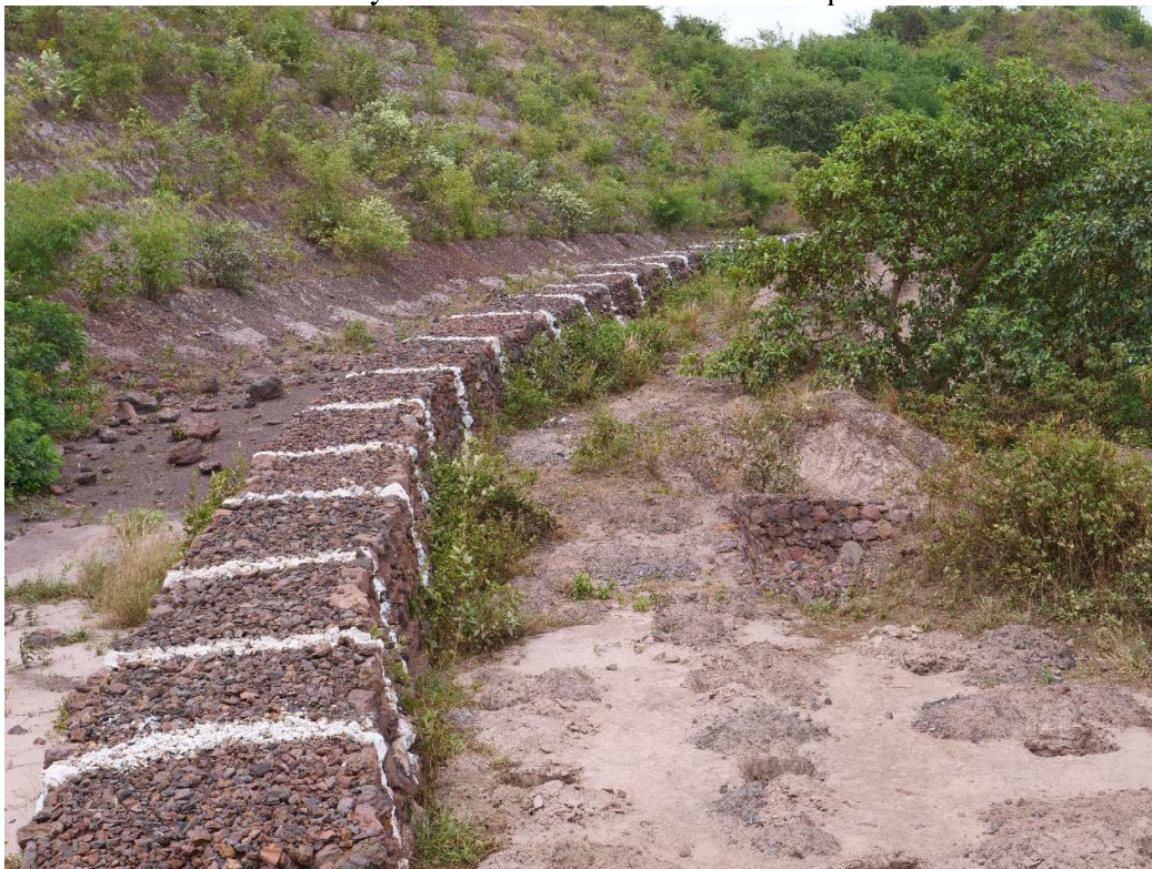
Toe Wall built below the dump at Dabaxikolla Mine
