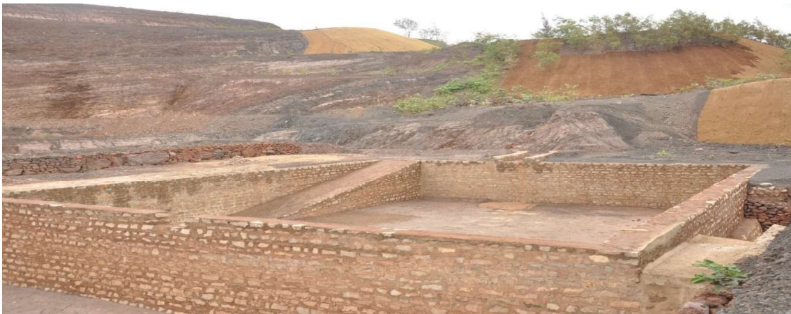
Silt Settling tank constructed at Governor Point Mine pit
