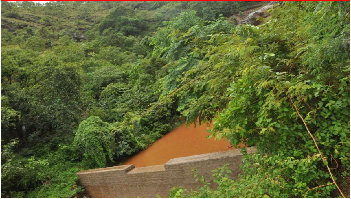
Stone Masonry check dam at Deogiri Section
