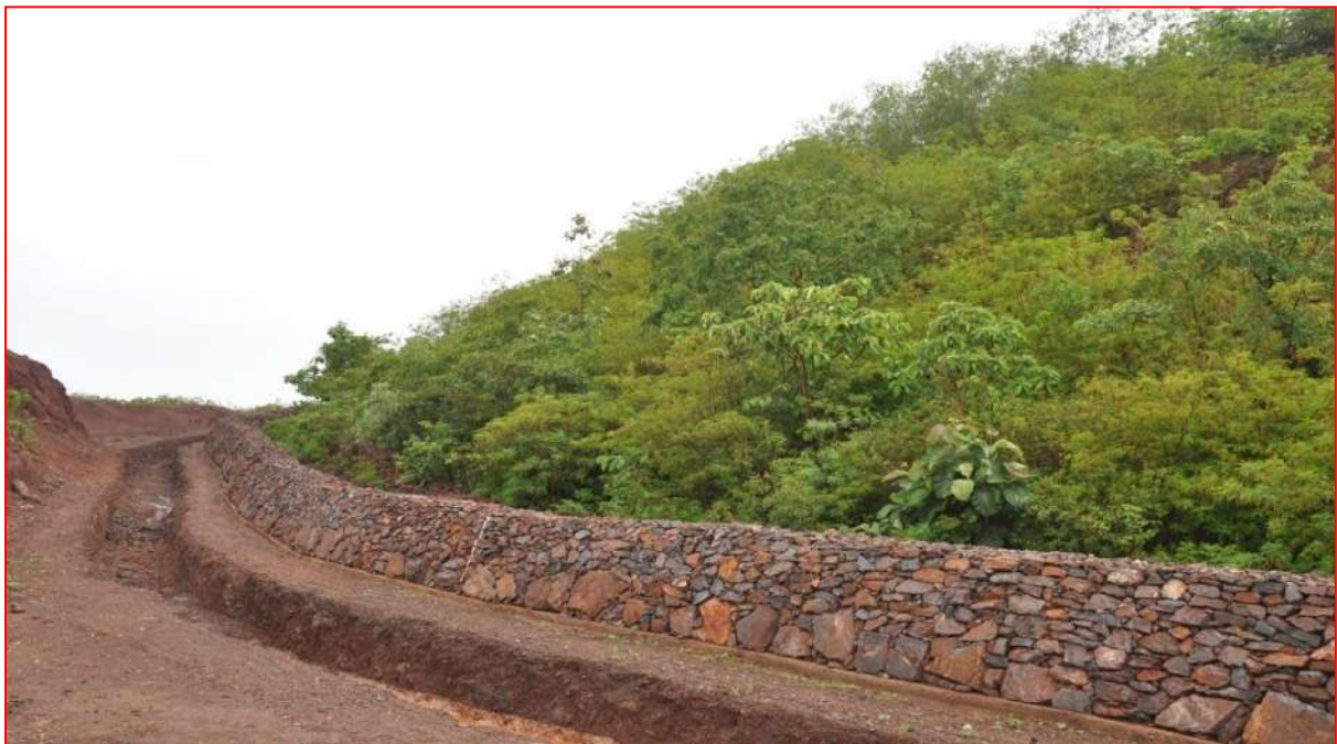
Garland drain along toe of waste dump
