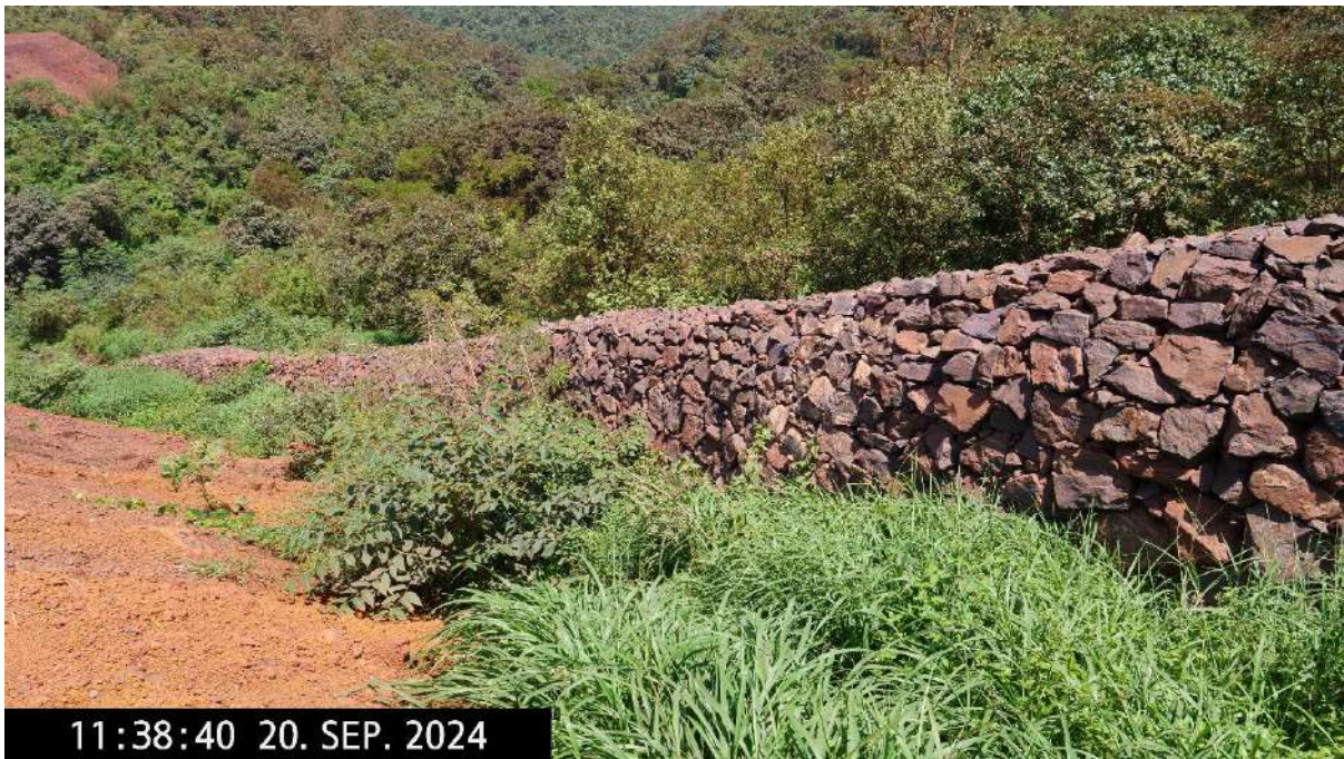
Toe wall at Kanivehalli Iron Ore Section of Subbarayanahalli
