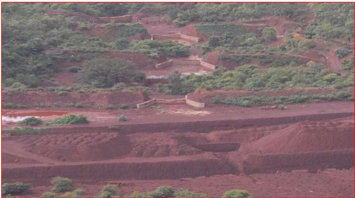
Series of Stone Masonry Check dam at KBHBG Section in Subbarayanahalli
