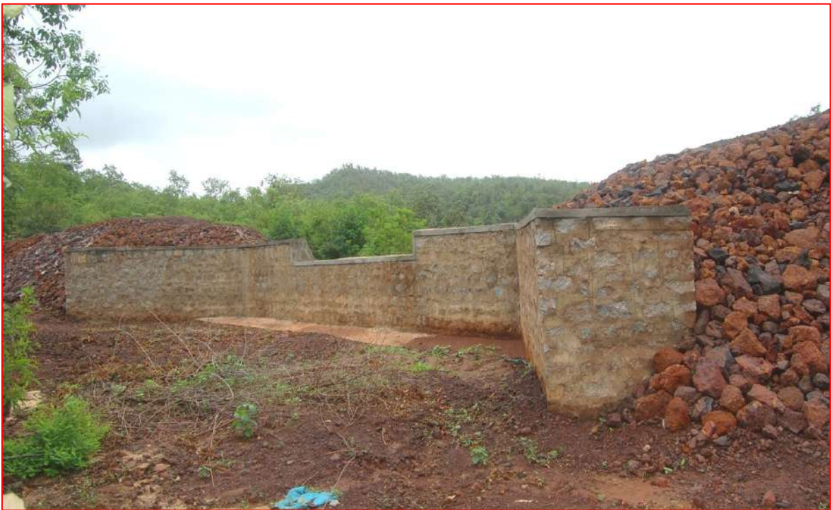
Stone Masonry check dam at Subbarayanahalli Section
