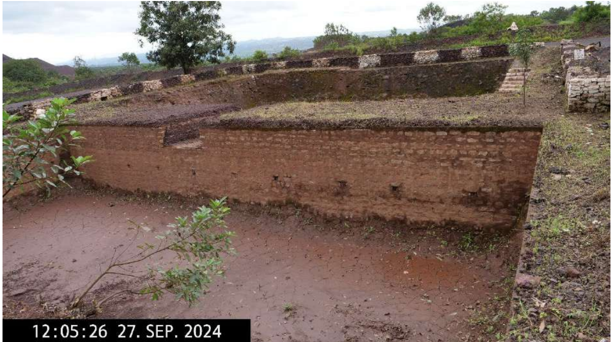
Cleaned Silt Settling tank and Rainwater harvesting tank at CBG Section, Deogiri
