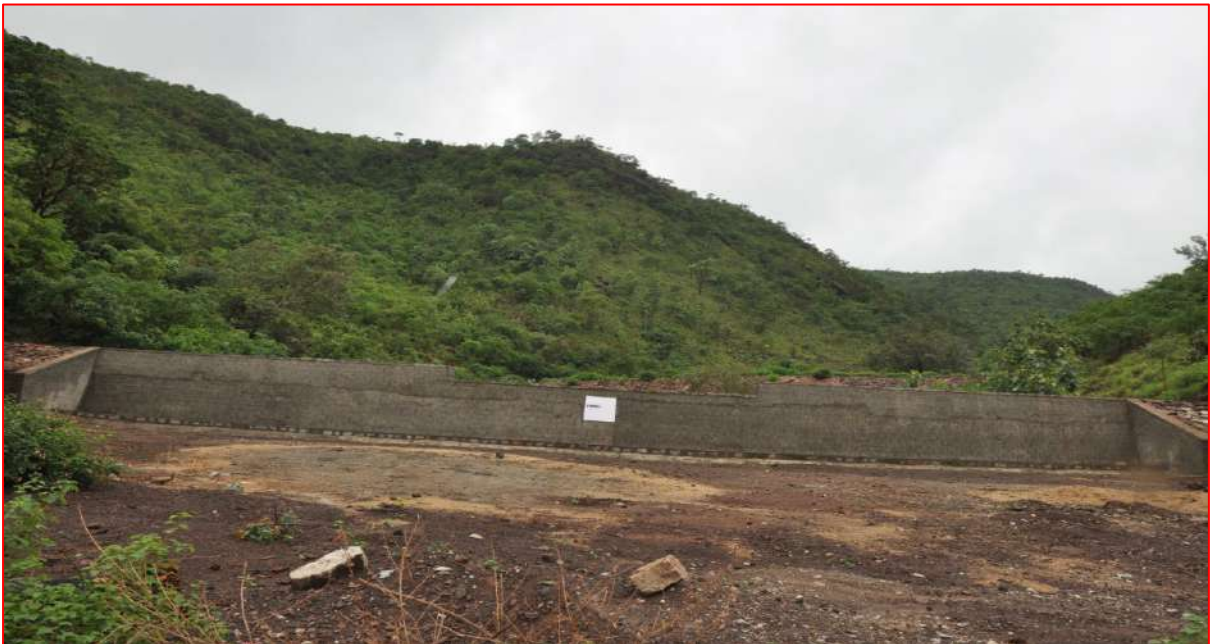
Stone Masonry Check dam at RMK section in Deogiri
