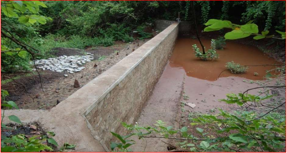
Stone Masonry check dam at Subbarayanahalli Section
