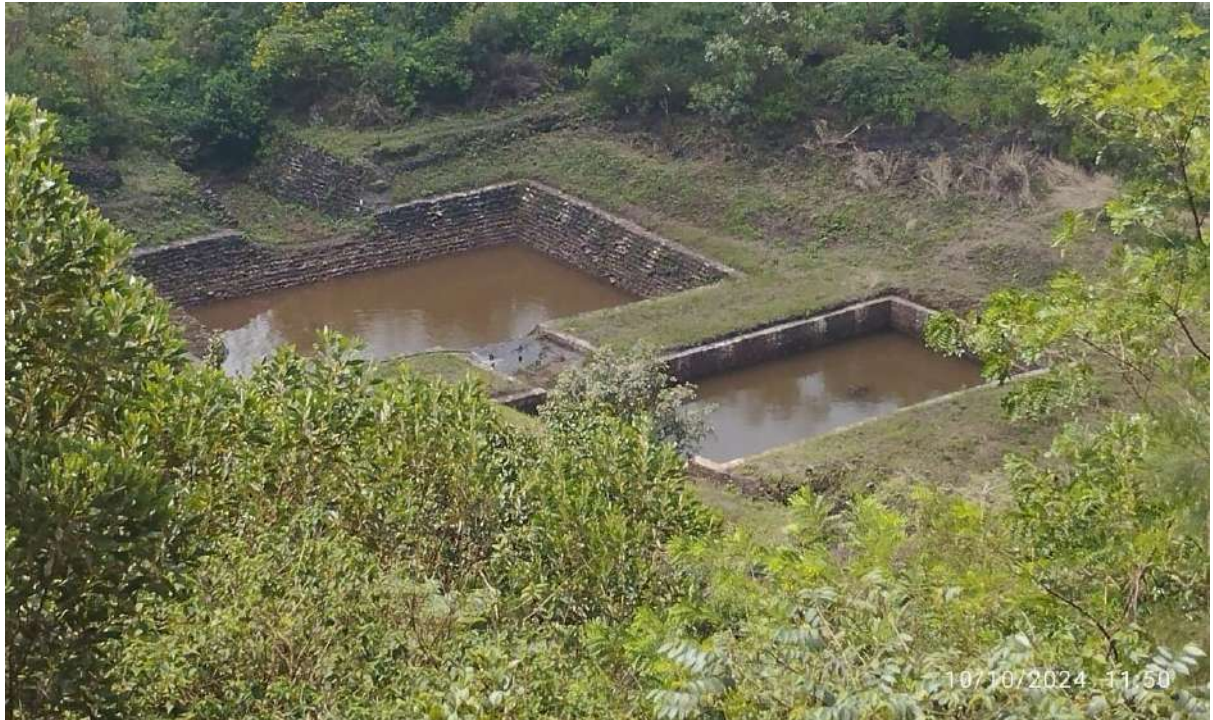
Water accumulation in Silt Settling tank and RWHP
