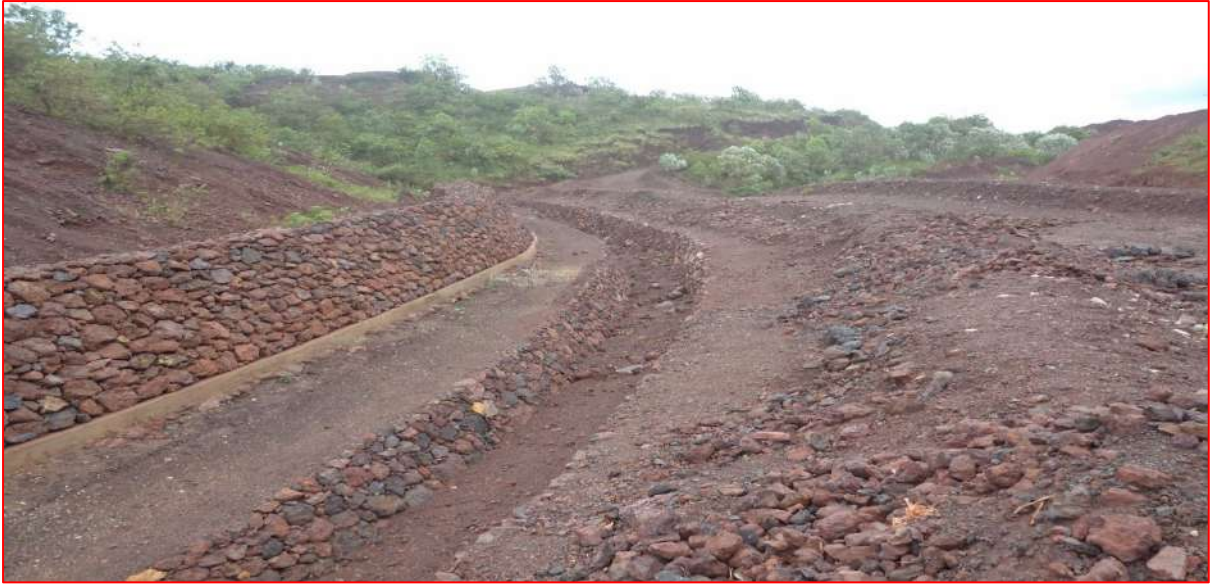
Stone pitched garland drain along toe of waste dump
