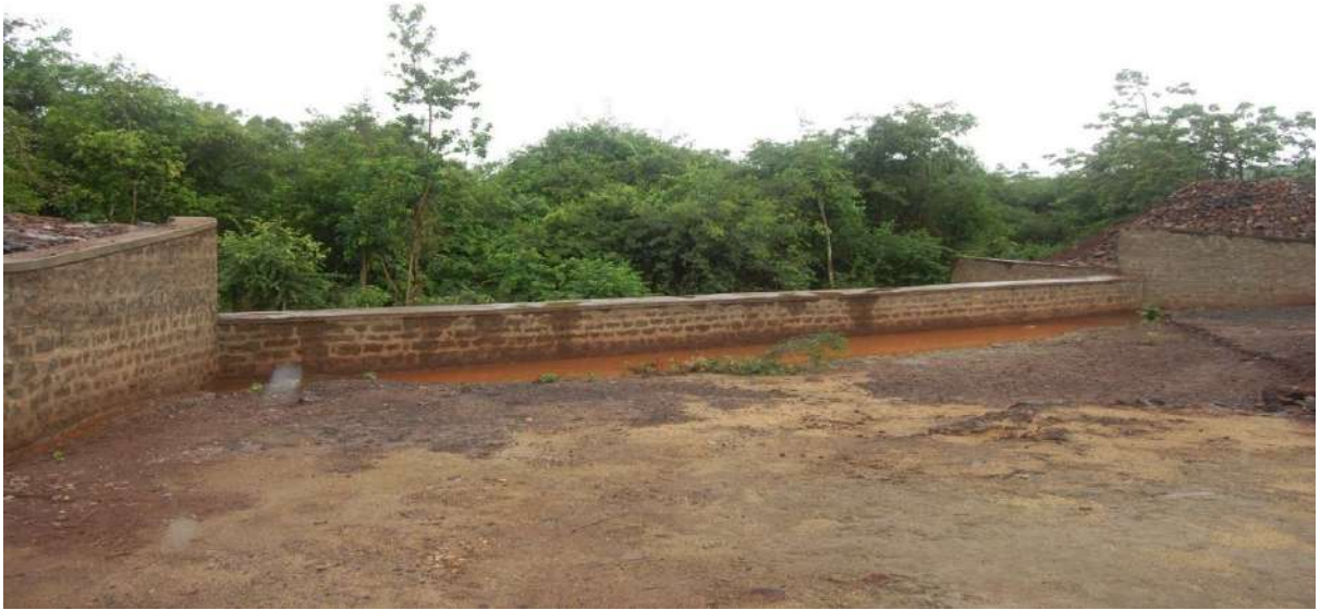
Stone Masonry Check dam at ML No 2678
