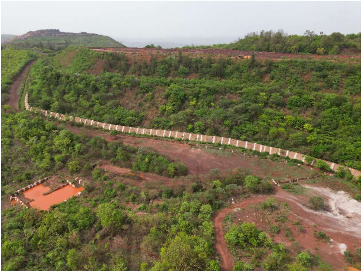
View of Stabilised waste dump with engineering measures at Kammatharu Iron Ore Mine
