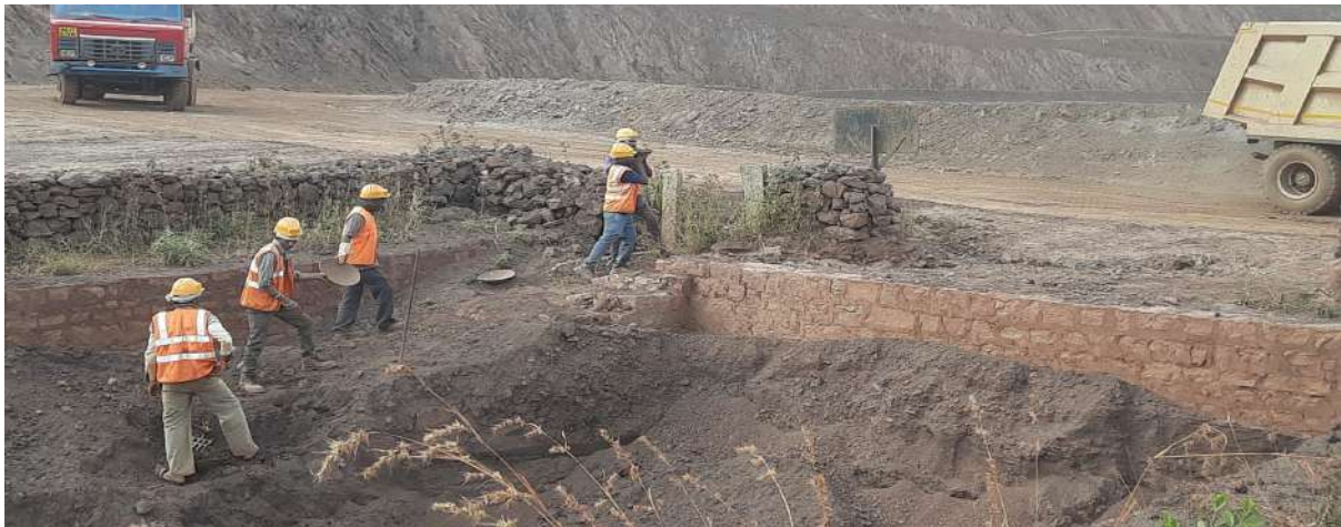
Manual De-silting of Silt Settling tank
