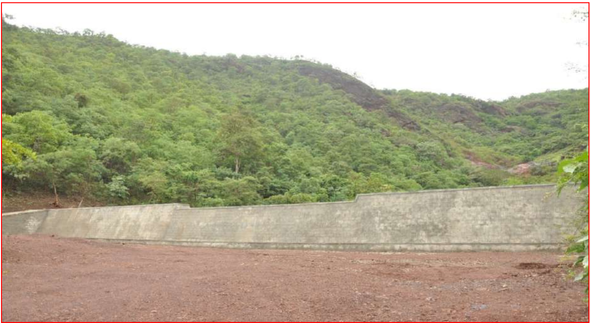
Stone Masonry check dam at Deogiri Section
