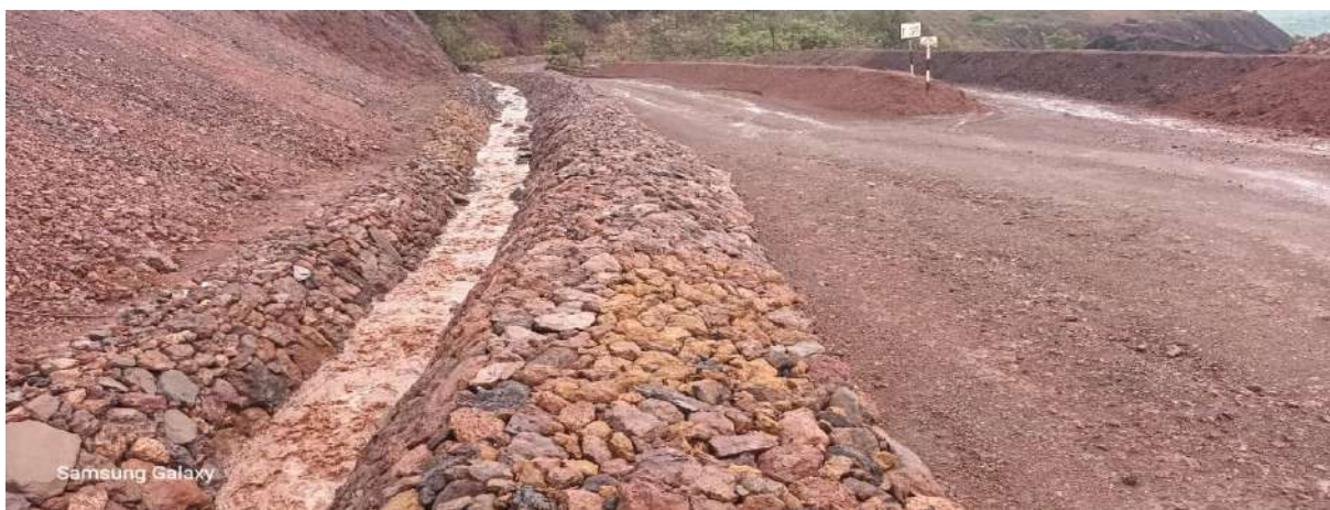
Rain water flowing through Garland drain at Mines
