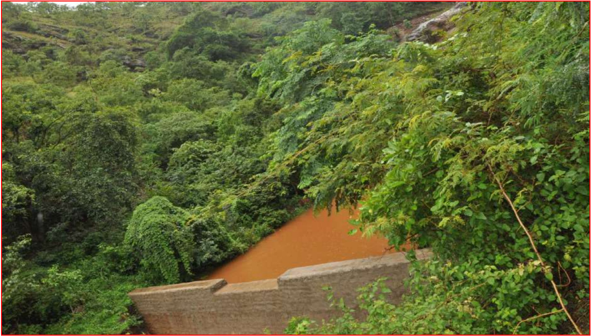
Stone Masonry Check dam at RMK section in Deogiri
