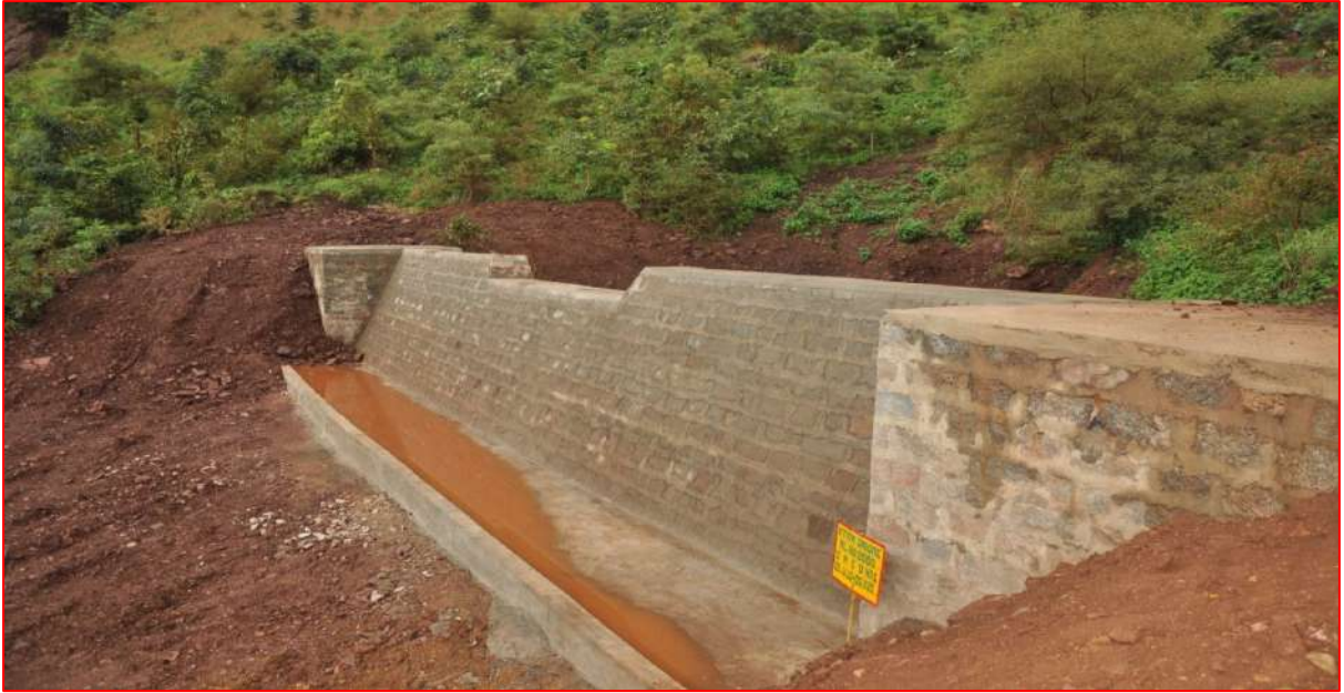
Stone Masonry Check dam at Kammatharu Iron Ore Mine
