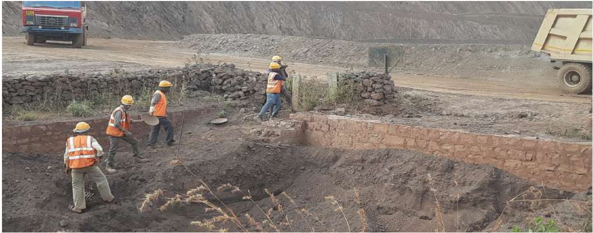
Manual De-silting of Silt Settling tank
