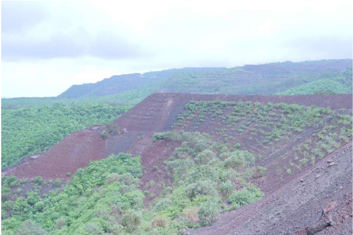
Implementation of Bio-Engineering measures for Dump Management
