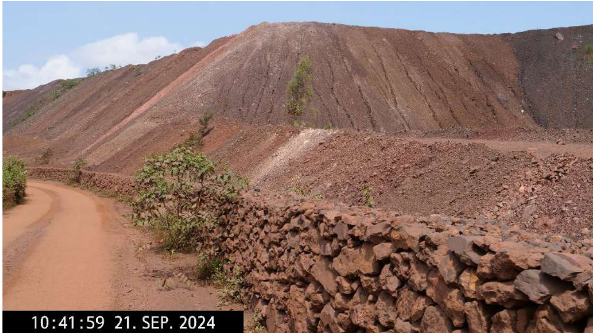
Toe wall built at CBG Section in Deogiri
