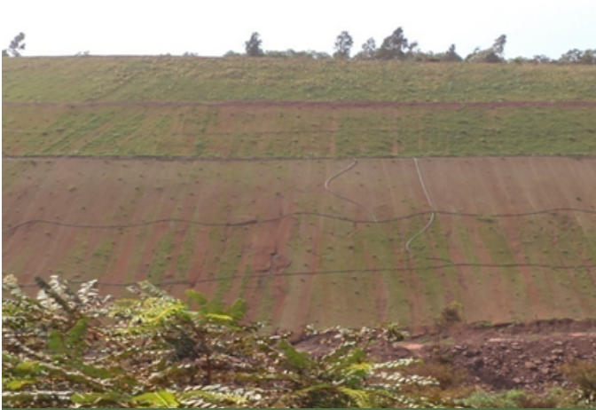
Coir Mat laid for stabilisation of Waste Dump
