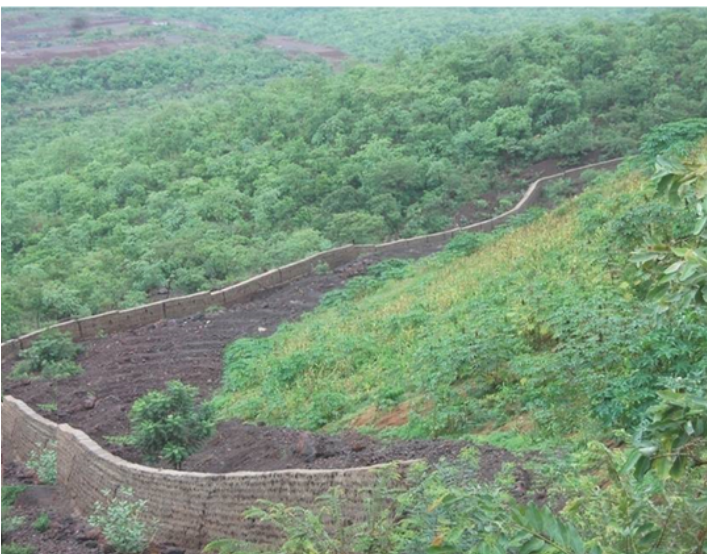
Implemented R&R Structures- Masonry toe wall for the waste dump
