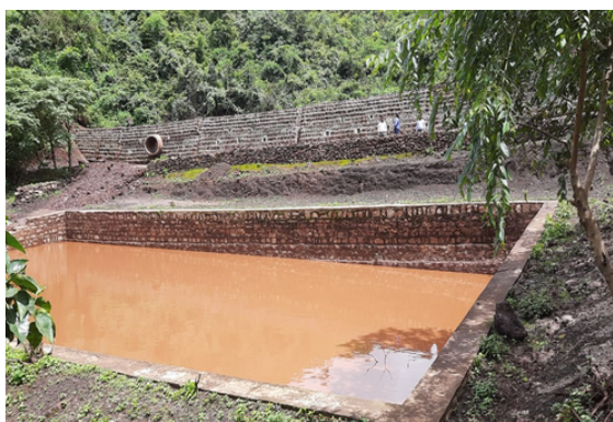
Implemented R&R Structures- Silt settling tank
